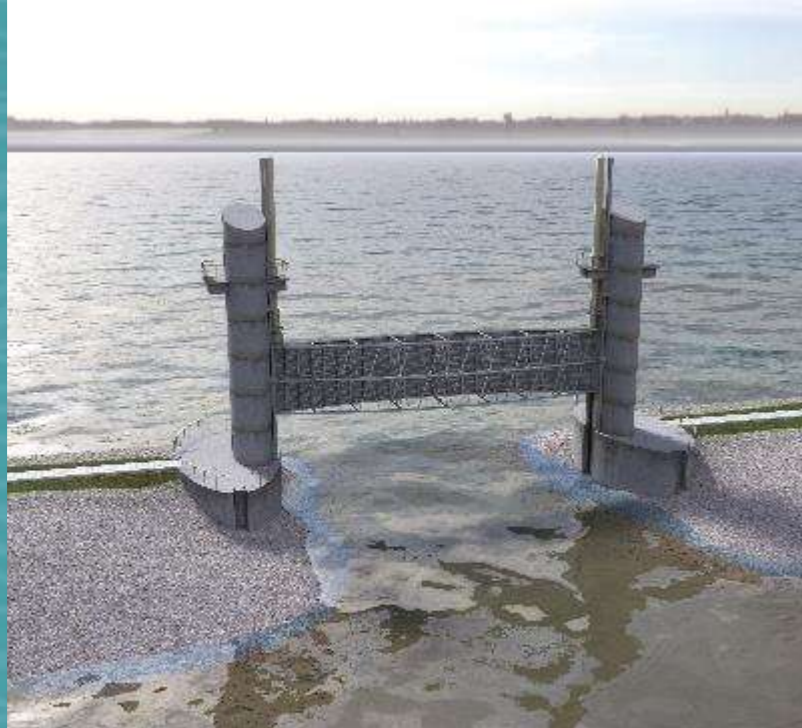
Open vertical lift gate
