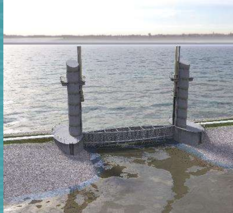
Closed vertical lift gate
